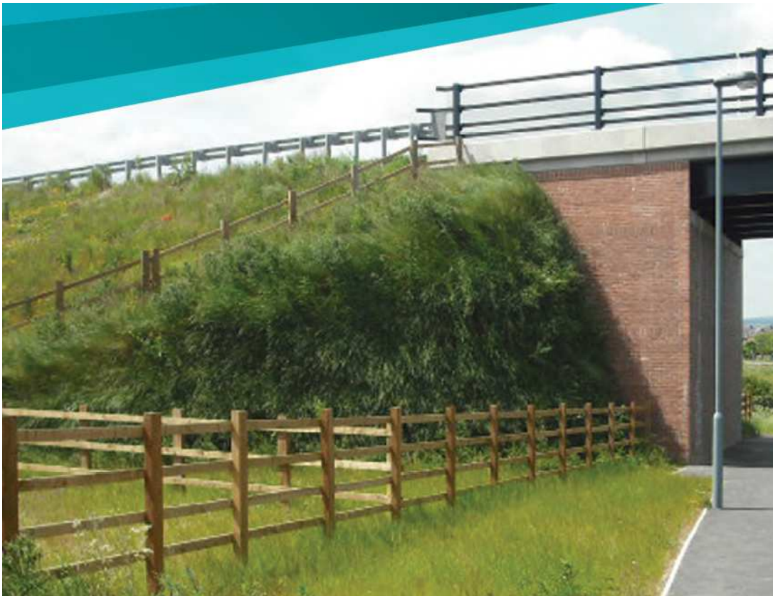
Figure 1 – Indicative detail of reinforced earth embankment (note that the bridge abutment remains as reinforced concrete, not brick as shown above)
